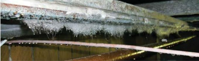
Mold growth visible on a floor joist caused by a burst water pipe.
