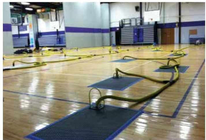
Single Source's Floor Drying System for hardwood floors
